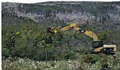
Clearing Access Road
