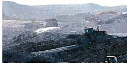
Plant Site Leveling
