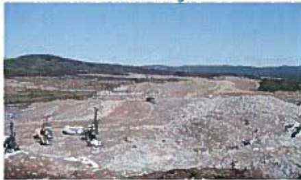
Main Plant Site
