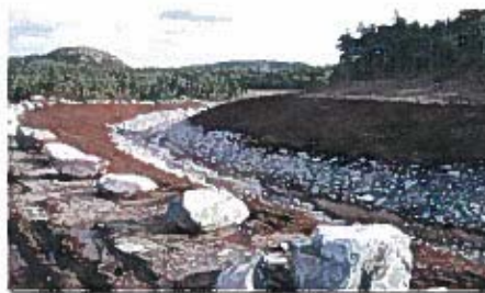
Storm Water Diversion Channel
