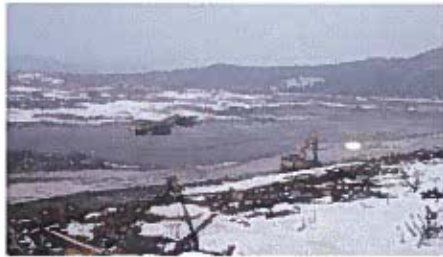
Placing Fill at Neutralization Building Area
