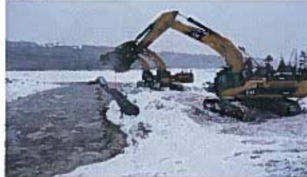
Intake pipe installation for Camp Water Supply
