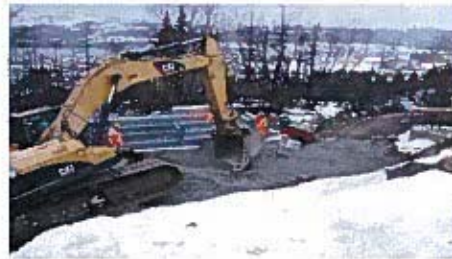
Bin Wall Installation
