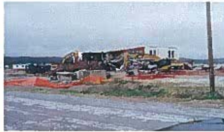
Demolition of Administration Building
